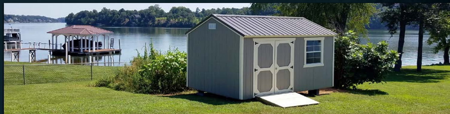
CLAY PAINT & NAVAJO TRIM PAINT ON LP SMART PANEL SIDING
