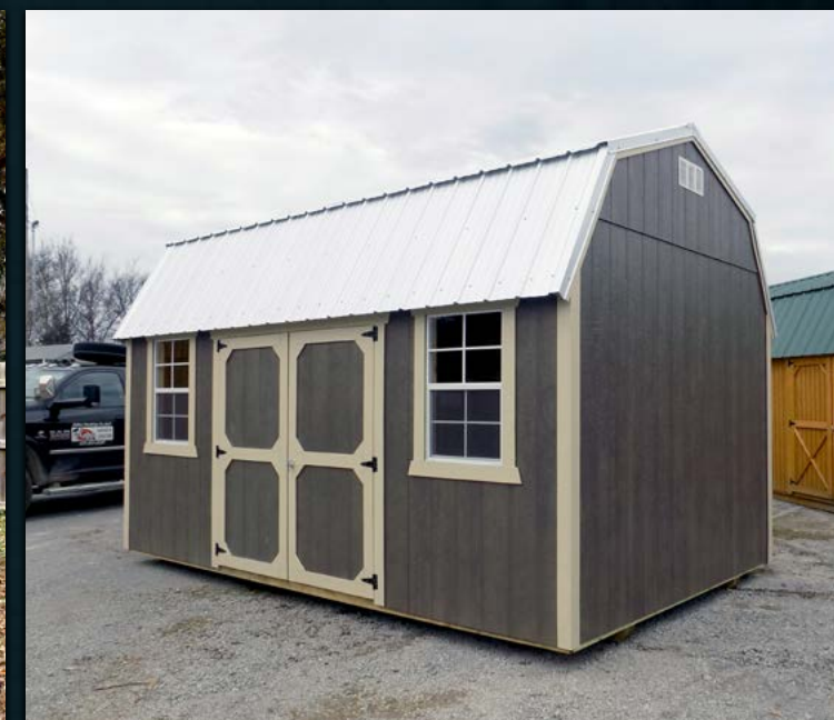
DRIFTWOOD URETHANE & BEIGE TRIM PAINT ON LP SMART PANEL SIDING
